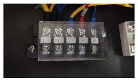
Note: In the case of three-phase models, swapping two phases may cause the electric motors to run in the reverse direction, which can lead to damage. For this reason, the unit has a built-in protective device that breaks the circuit if the connection is not correct. If the red LED above this safety device lights up, **you must swap the connections of two of the phase wires**.
